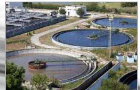
Water & Wastewater Treatment
